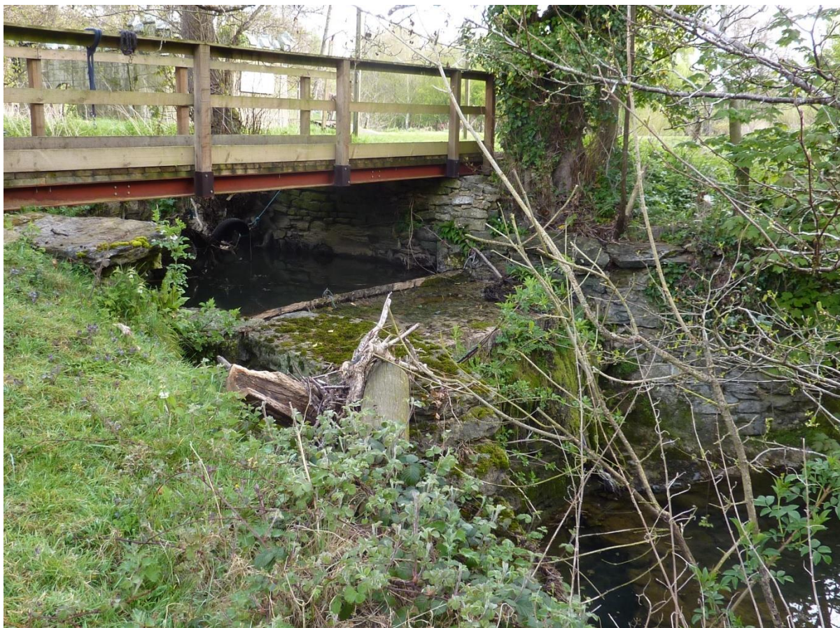
Figure 2: The Island weir: impassable to fish at all flows, and allowing almost no water into the main channel of the River Brue through the Gants Mill estate at the time of this visit
