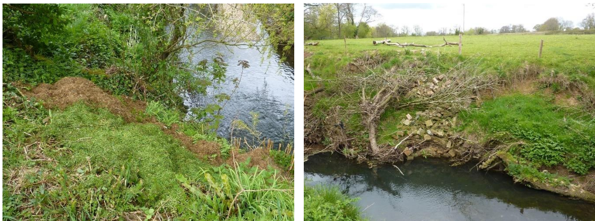
Figure 19: Disposal of grass clippings (left) and builder's waste in a counterproductive attempt to protect the bank (right) on the river banks should be avoided
