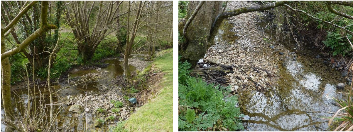
Figure 8: Subsurface tree roots provide cover for fish as well as 'forcing' scour and deposition; note the tree root structures still helping to reinforce the RB, although this also seems to be grazed and would benefit from fencing and revegetating (including targeted tree planting for future hinging down into eroded areas of bank)
