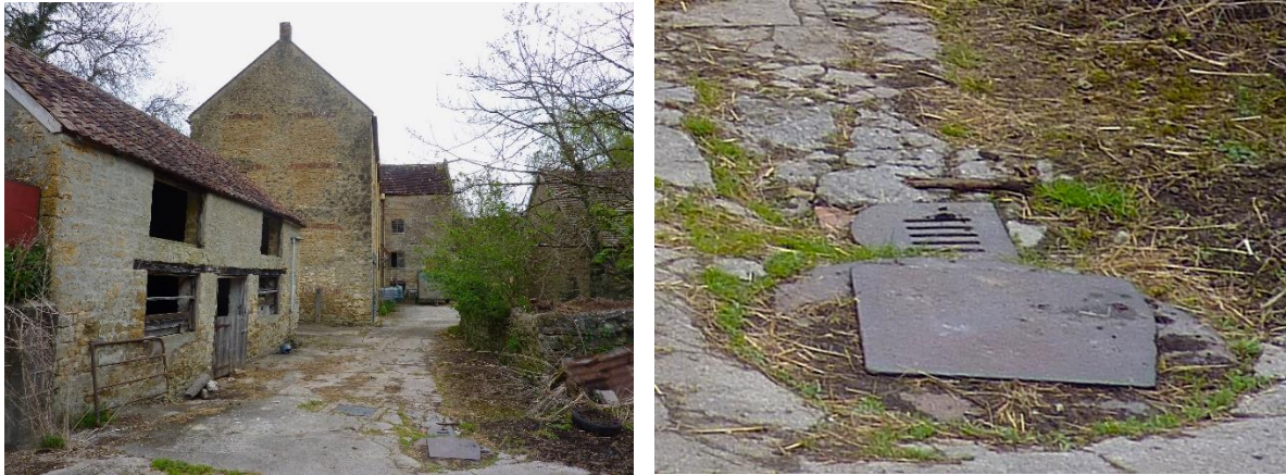
Figure 10: Gants Mill buildings being used for agricultural purposes; the cast iron drain grate could carry contaminated water directly into the river
