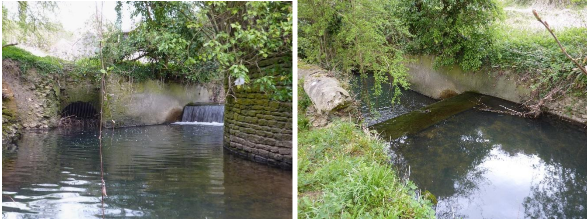
Figure 9: Views of Farm weir from downstream (left) and upstream (right)
