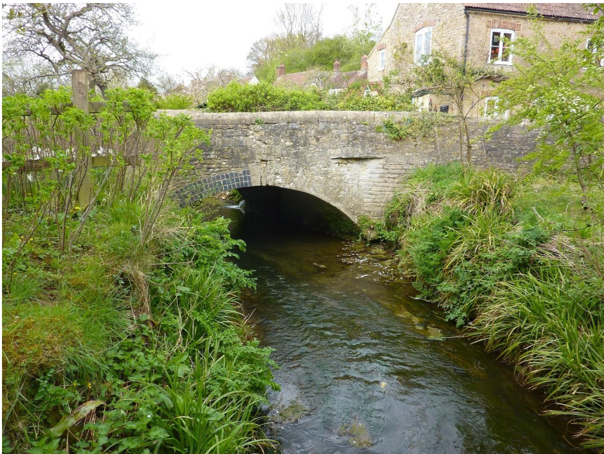
Figure 2: Pitcombe bridge, viewed from the gardens upstream
