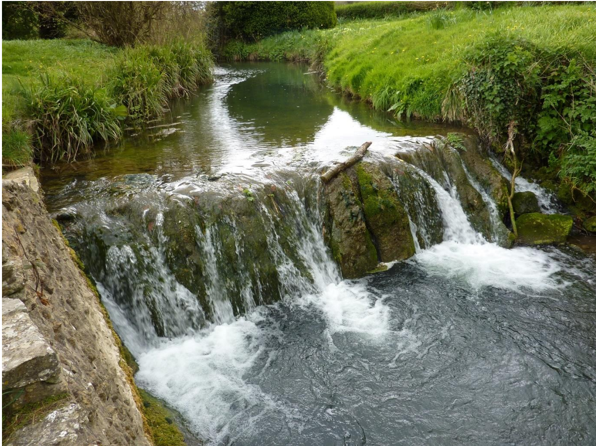
Figure 14: Cole Manor gardens weir: smaller than the head weir, but still an obstruction to fish passage and sediment transport
