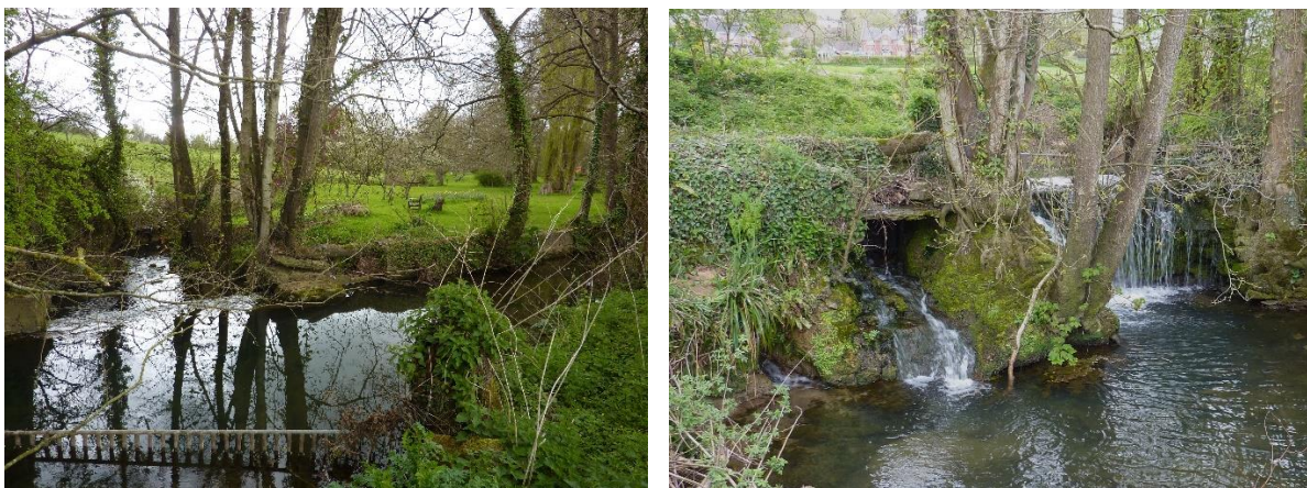
Figure 9: Cole Manor Mill head weir, seen from upstream (left) and downstream (right): a barrier to fish passage despite being in a state of disrepair. The pool below the weir offers habitat for adult trout, but the weir will block any efforts to migrate upstream
