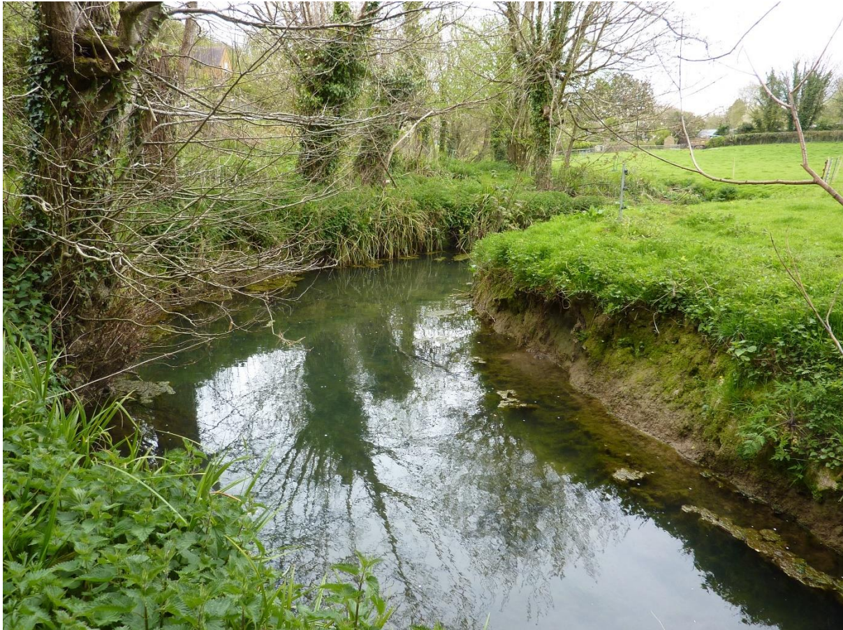
Figure 7: Looking upstream from ST 67147 33216: the river's RB is recovering some of its trailing vegetation following historic 'stream clearance' and dredging, but the square-profiled LB still lacks vegetation, partly due to grazing, and continues to be subject to block failure. Fencing off a 5-10m buffer strip, and perhaps regrading the angle of the bank, will help to ensure that the LB landowner will not continue to lose land to excessive erosion in future.
